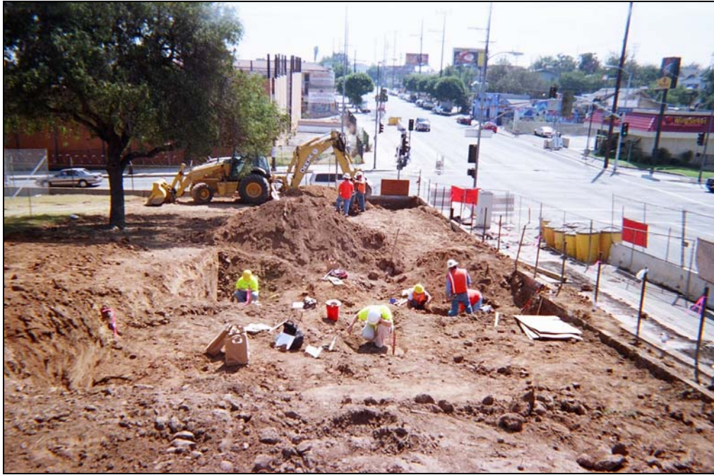
Figure 2.5. Area C archaeological exploration with redirected heavy machinery testing
