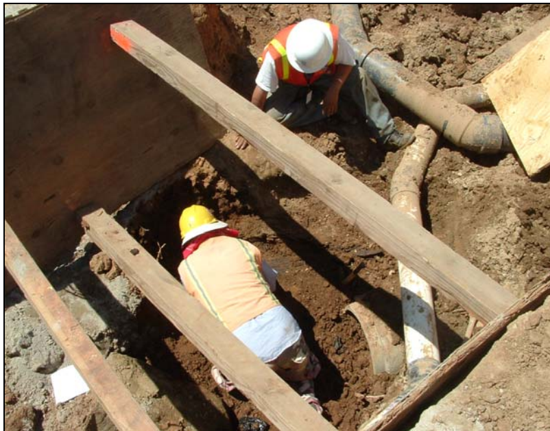
Figure 2.7. Excavation of recovery in the pipe trench
